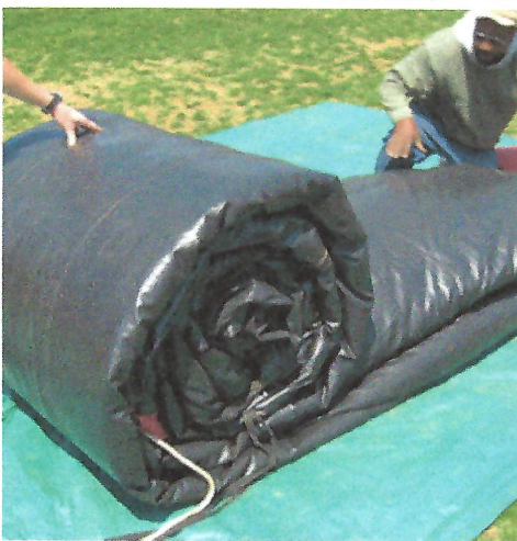
Step 9-10: Tuck in Ports (Blower tubes) and tie off roll.
