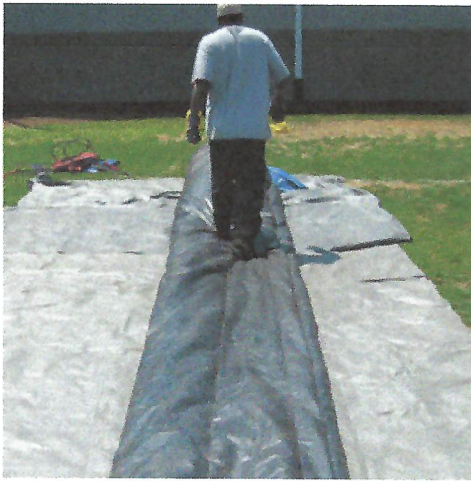
Step 2-6: Fold the Inflatable in 2-3 feet lengthwise and walk out air towards Ports (Blower tubes).
